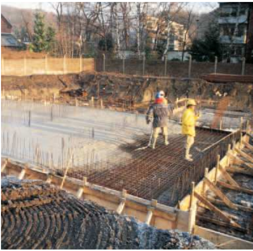
DELTA®-MS Sub-base Course will bear the weight of workers and wheelbarrows, saving time and money.
