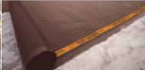
Overlaps should be 20 cm minimum.
