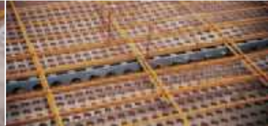
Reinforcement-mesh spacers are safely held in place.
